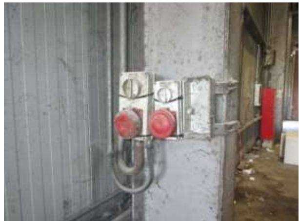
Image 51 – damaged 3-phase power sockets
