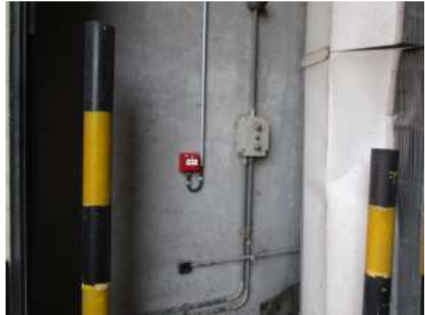
Image 59 – manual call point sign missing
