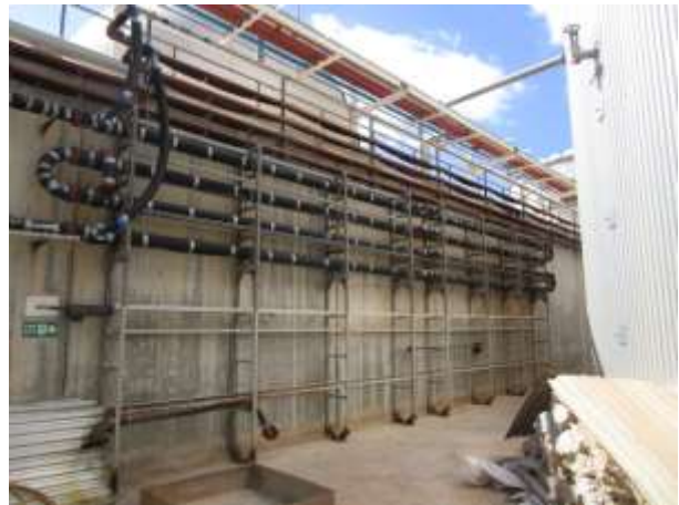
Image 61 – no labelling on pipework
