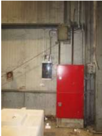
Image 58 – no signage on fire cabinet or electrical distribution board
