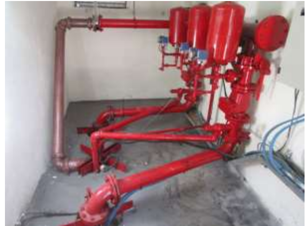
Image 69 – submersible fire pumps
