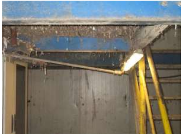
Image 53 – damaged electrical lighting installation
