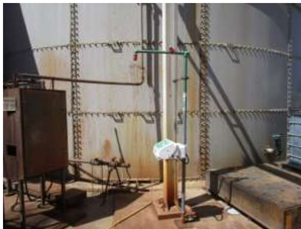
Image 39 – emergency shower in the vicinity of the acid storage in the tank farm area
