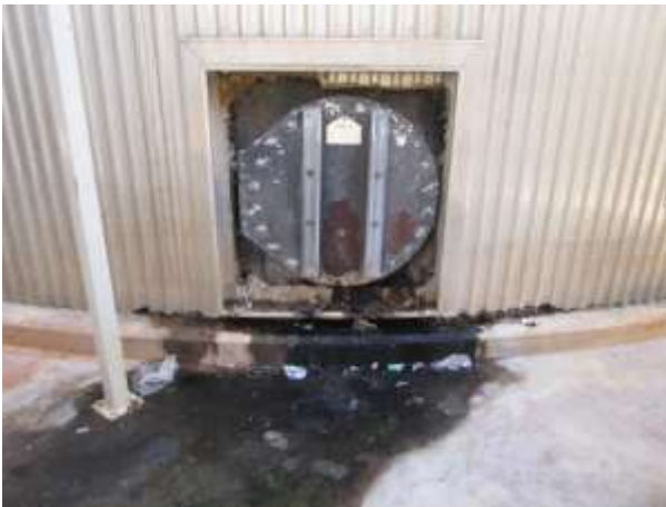
Image 60 – confined space entry, no permit to work signage
